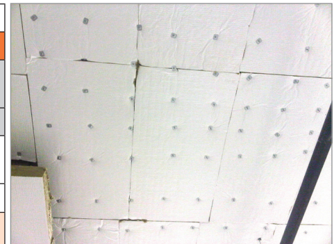
Over used stick pin installation. This increases the thermal bridge and reduces thermal efficiency.
