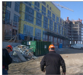
Exterior walls - Insulation to steel stud
