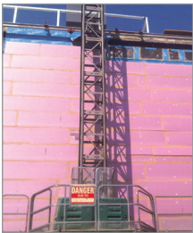
Exterior walls - Insulation to concrete
