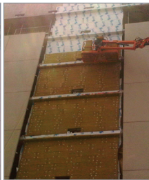
Exterior walls - Insulation to concrete
