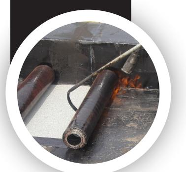
When used with a cap sheet, **Torchflex TF-95-SF-Base** satisfies the requirements of CGSB-37.56-M, as well as ASTM D6163 for Type I, Grade S materials.
